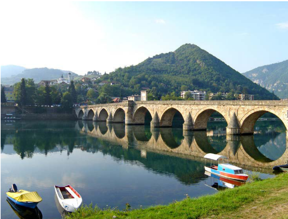
Figure 10: The Mehmed Paša Sokolović Bridge in Višegrad across the Drina River in the east of Bosnia and Herzegovina was built at the end of the 16 th century (source: Andrić Branislav).
