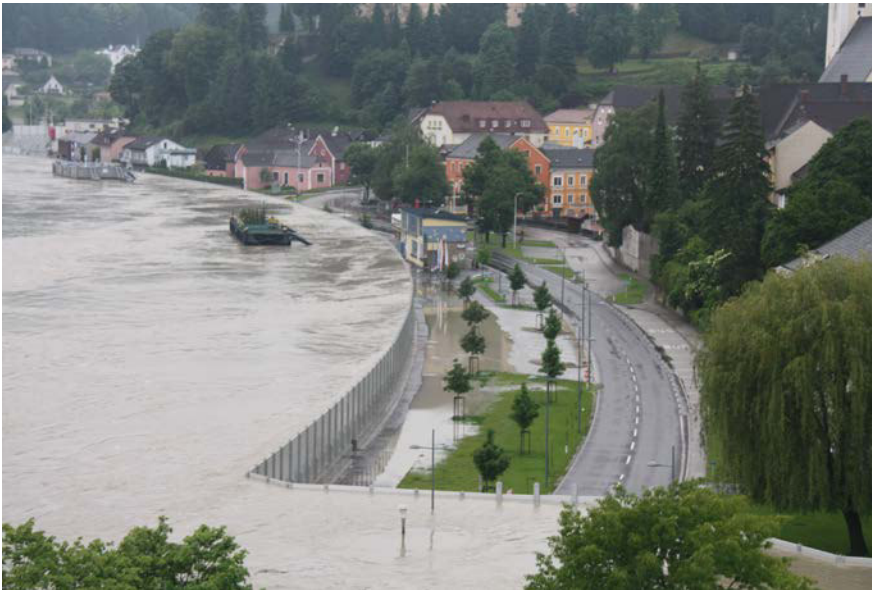
Figure 3: Mobile flooding protection structures such as those in Grein (Wachau) on the Austrian Danube can increase flood peaks and inundation risk downstream (source: Robert Zinterhof)
